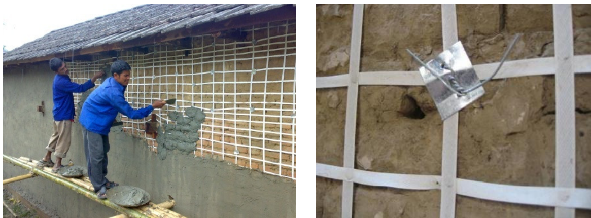
Fig 3.5 Implementation of PP band method of retrofitting in Kathmandu Valley (left) and anchorage throughout the wall (right)
